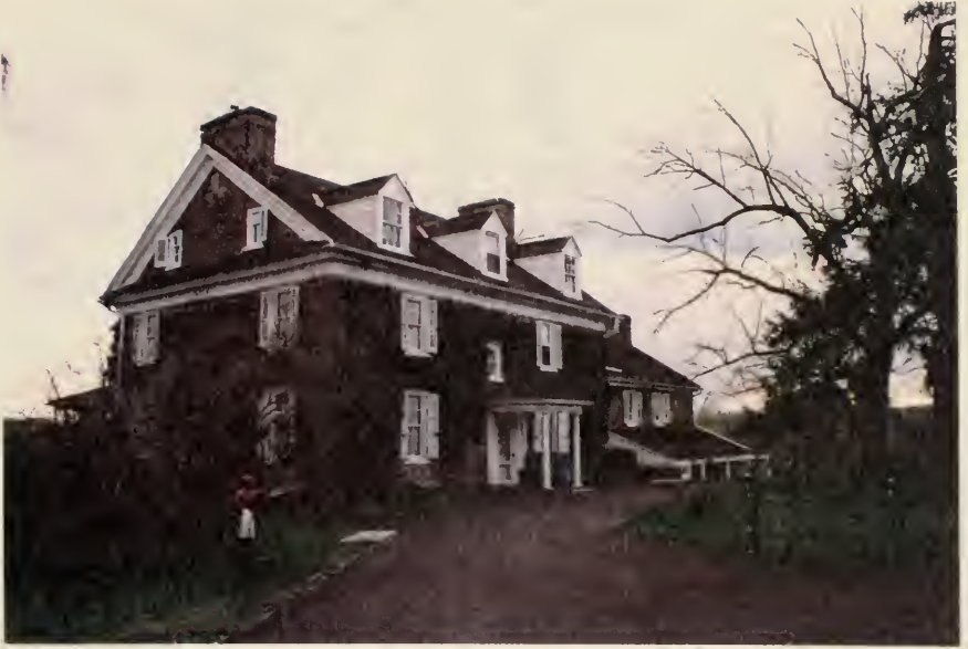
Figure 8. Mill Grove Mansion, existing appearance of north and east elevations. (1994)
